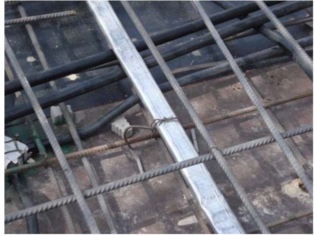
(c) Grouted slab construction
